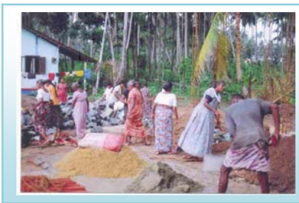
Community volunteering to set up Coir Processing Centre
