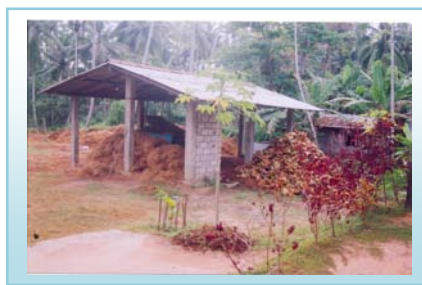
Coir processing Centre and the Machinery
